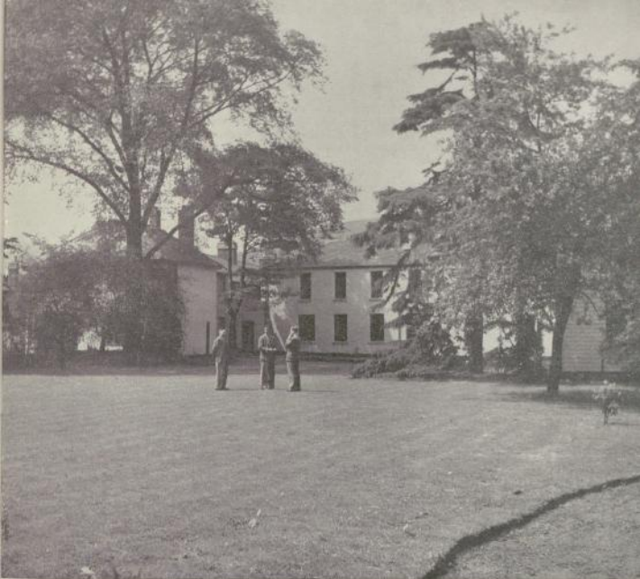
The New Settlement House at Risca.
